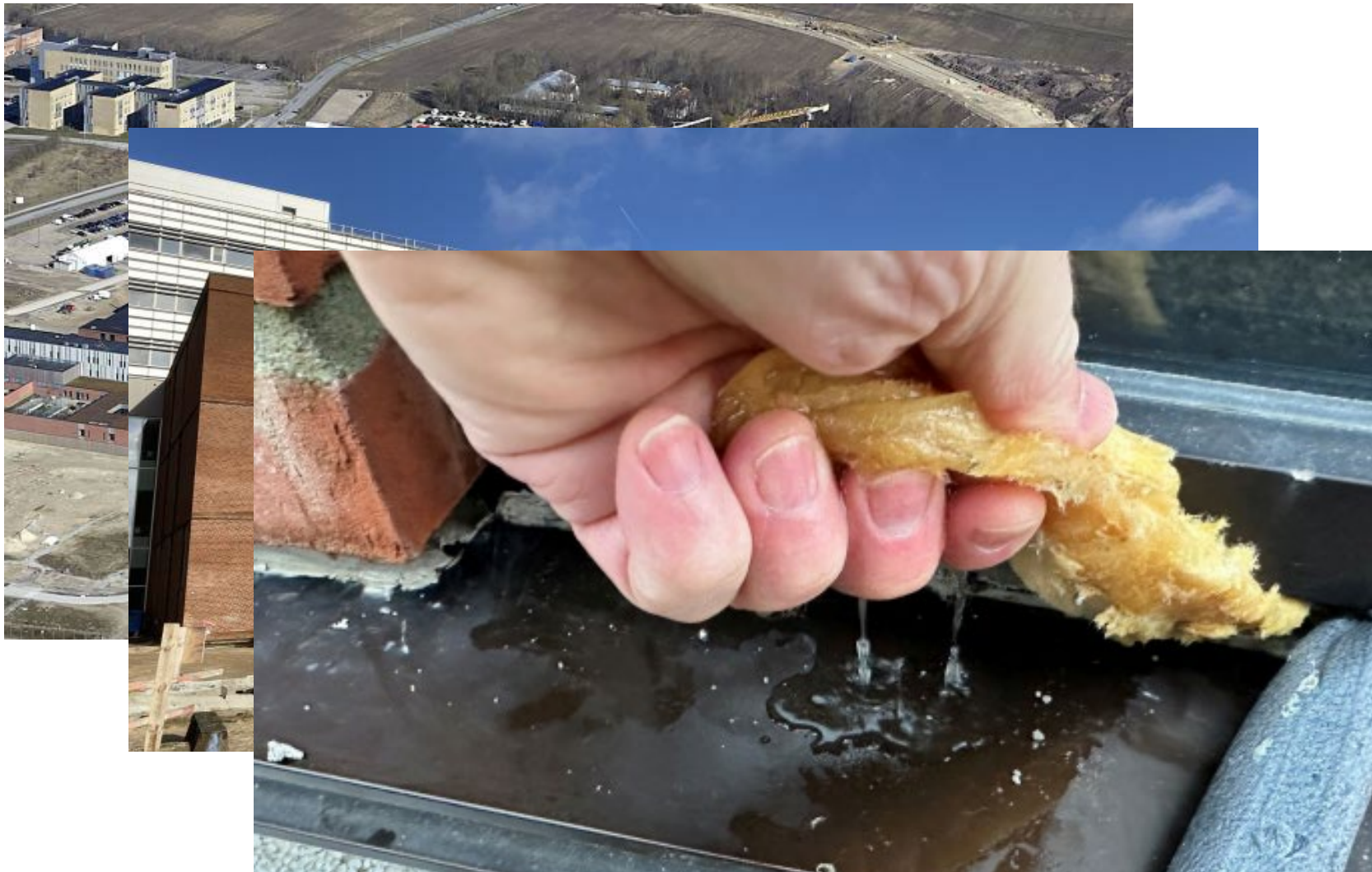
Pictures from Ingeniøren and Danmarks Radio
