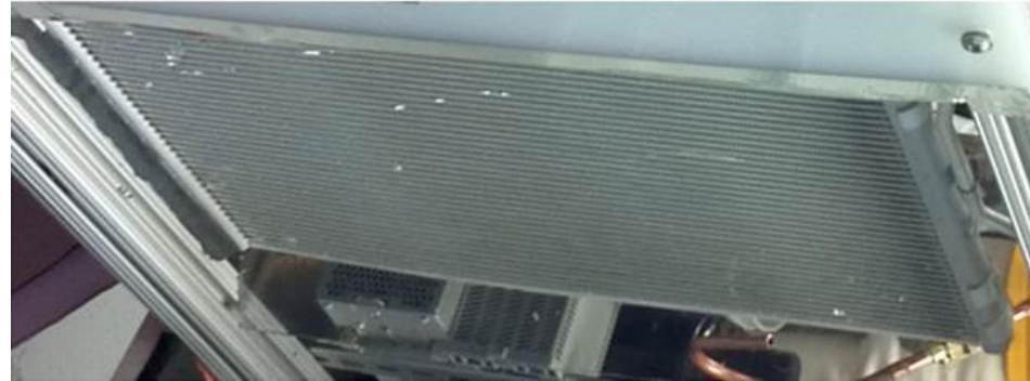
Micro-channel condenser
