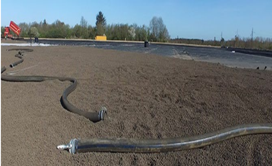
Floating insulation layer
